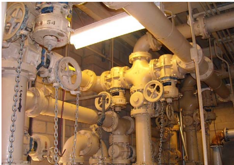
The City's water distribution system has more than 330 miles of water mains
